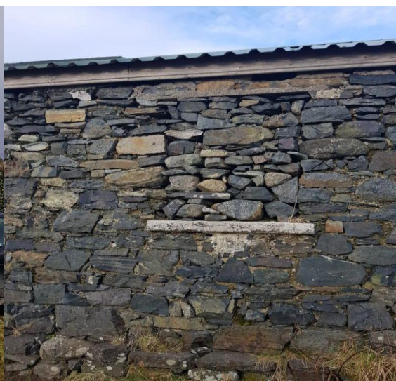
Window blocked with dry stone
